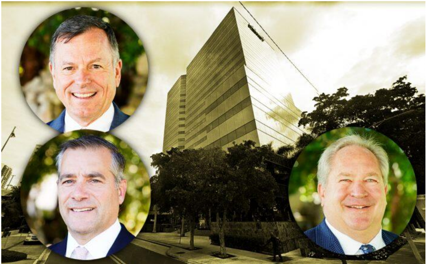
1 East Broward Boulevard in Fort Lauderdale and Pacific Coast Capital Partners' co-founders William Lindsay, Aaron Giovara and Donald Kuemmel (PCCP, Google Maps)
